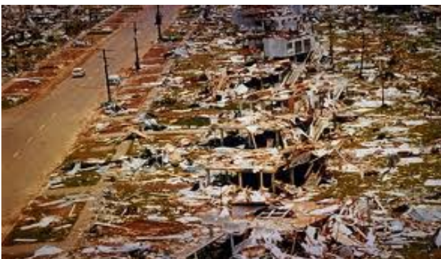
Figure 3: Example of damage - Cyclone Tracy (Source: BoM)
