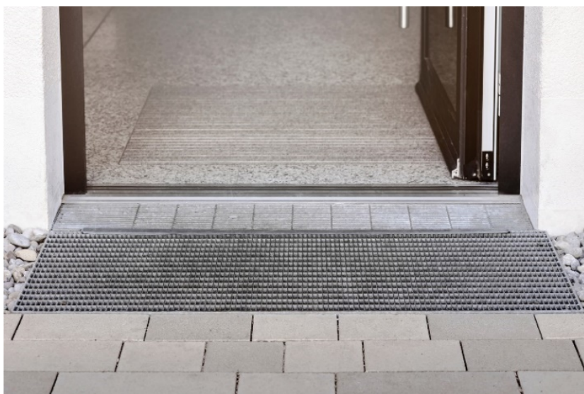
Figure 4.6 Channel drain at entrance door
